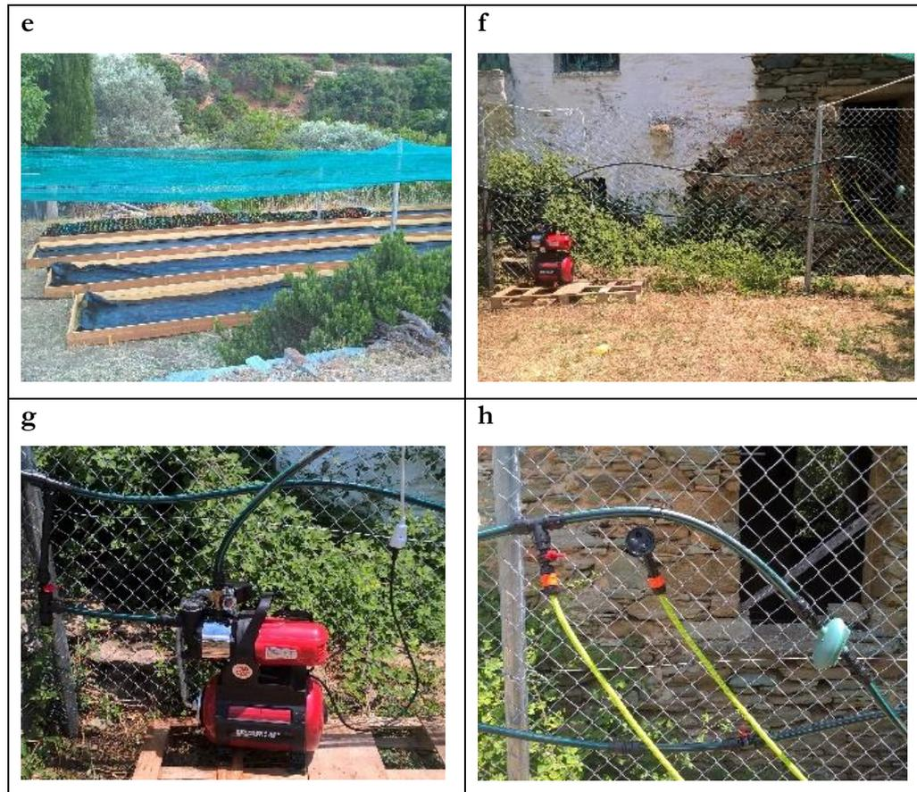
**Figure 2e)** View of the removable shadow net, **2f)** The irrigation infrastructure, **2g)** The water pump, **2h)** Detail of the watering programmer and the branching for manual irrigation.
